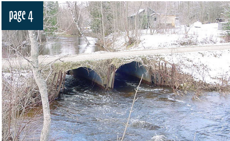
Problematic culverts on the Carp River.
