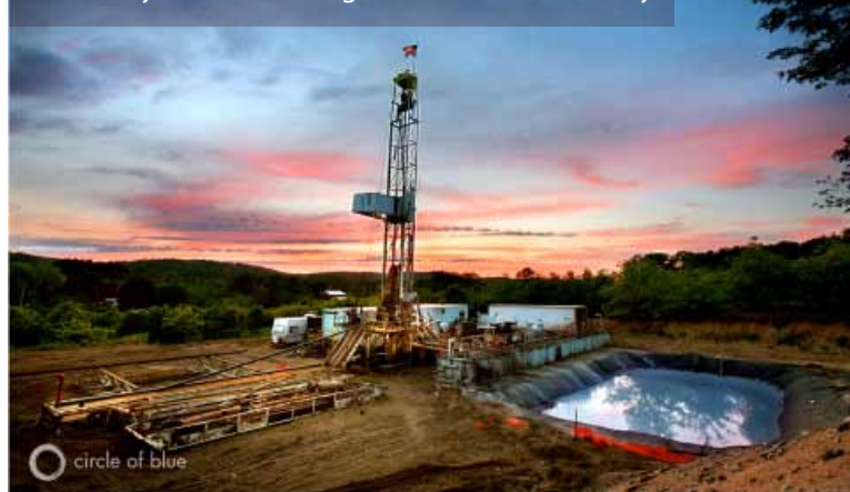
A recently drilled natural gas well in Benzie County.
