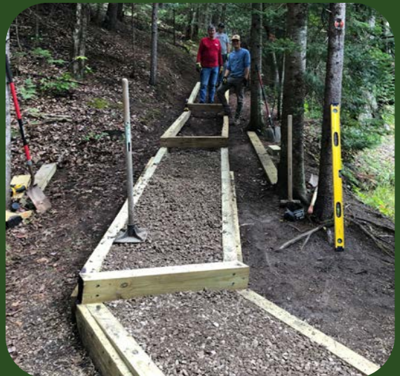
Above and below: This fall, Eagle Scout candidate, David Johnston (below right), and his Troop constructed a new staircase at the Agnes S. Andreae Preserve to prevent erosion and improve slopes for walking.
